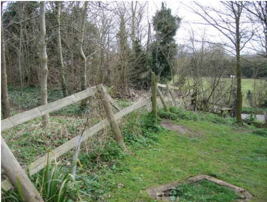
Damaged fence on the southern border
