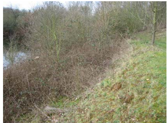
South Facing Bank
